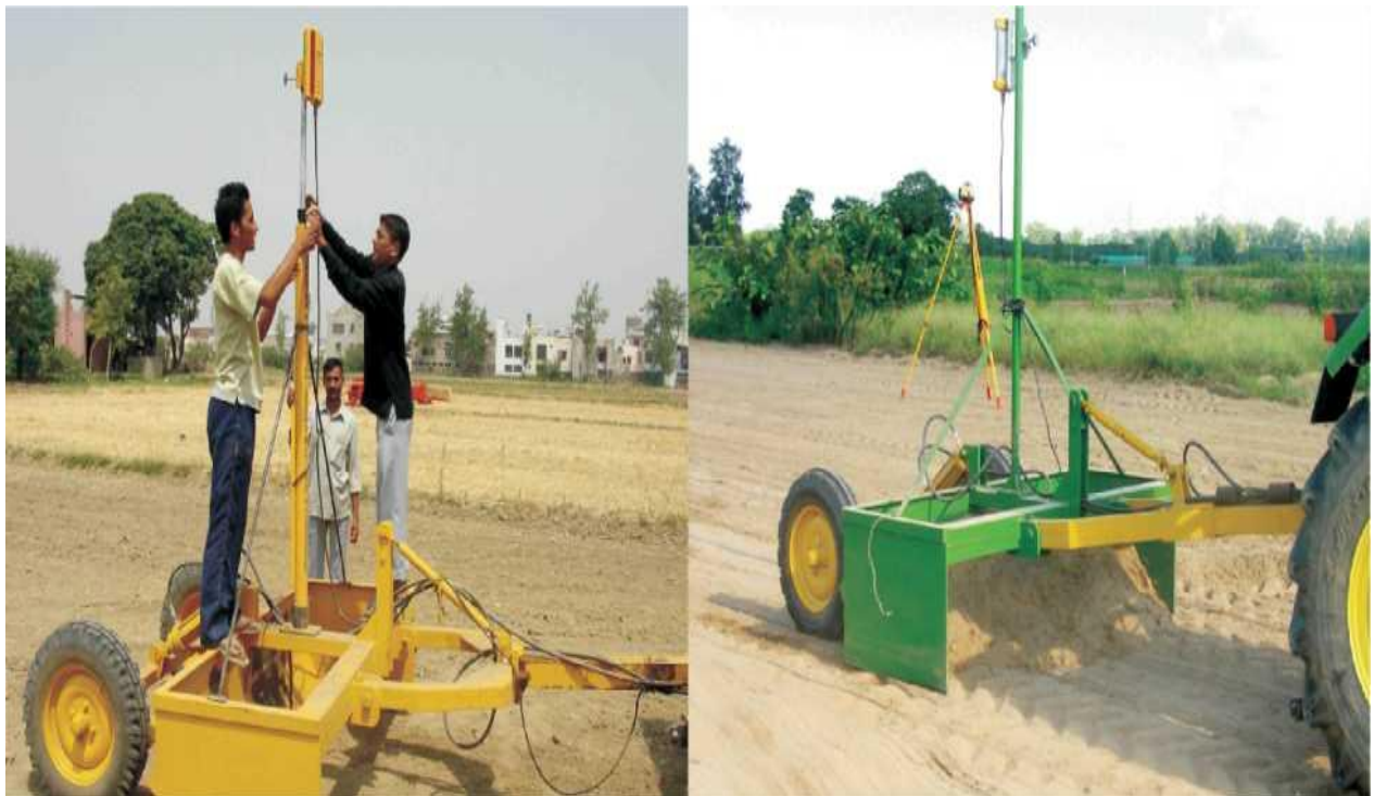
Fig. 8.3: Set the scraper blade and laser beam receiver at the location.
