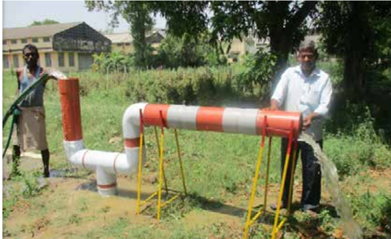
Groundwater recharge cum drainage unit tested
