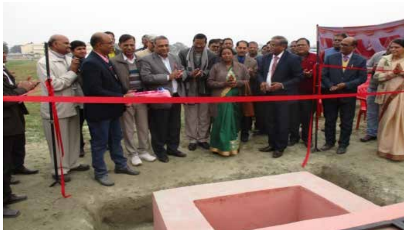
Groundwater recharge cum drainage unit inaugurated by Hon'ble Vice-Chancellor & Members of Board of Management on 25.01.2019
