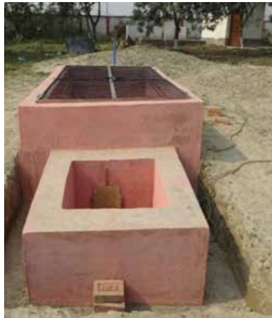
Plate 4.5.1. Groundwater recharge cum drainage unit installed in Pusa Campus
