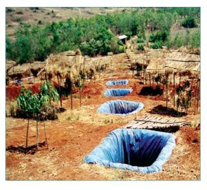
straw bundle (5 to 10 cm thick pre-lining cushioning bed) and HDPE lining film (500 micron). One Jalkund can hold 4000 litres of clean rainwater. Stored water in one *Jalkund* is sufficient to irrigate 10 mango or 20 cashew grafts during postmonsoon season of 30 weeks period (15<sup>th</sup> November to 15<sup>th</sup> June) @ 10 litres per
