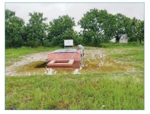
to waterlogged condition. There is no wheat sowing in most parts with late sowing in some parts of the village. As a result of installing the drainage cum groundwater recharge unit, excess water was drained out in the last week of November and timely sowing of wheat was possible after 20 years in Shri Mahto's field. Over 15 hectares and 10 farmers have been benefitted with this technology so far.
