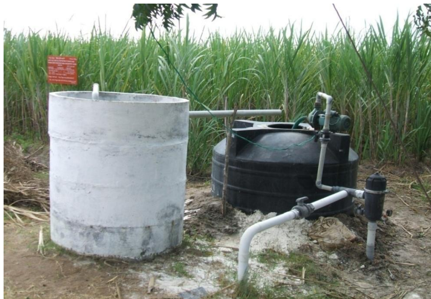
Plate 3. Gypsum bed treatment of alkali water
